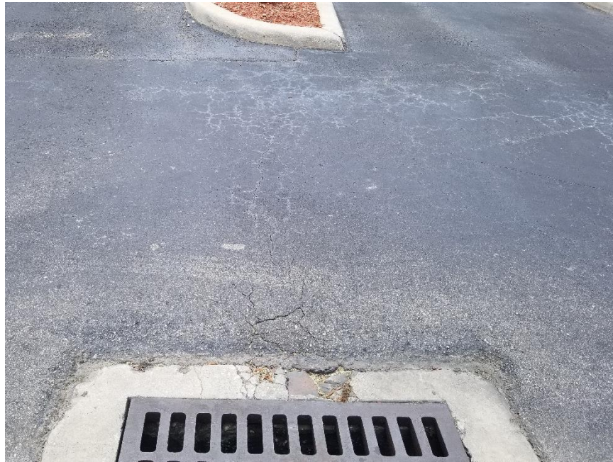
Alligator Cracking (Typical)
