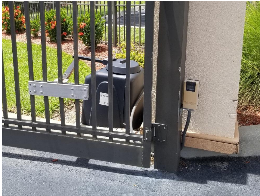
Motorized Opener (Typical)
