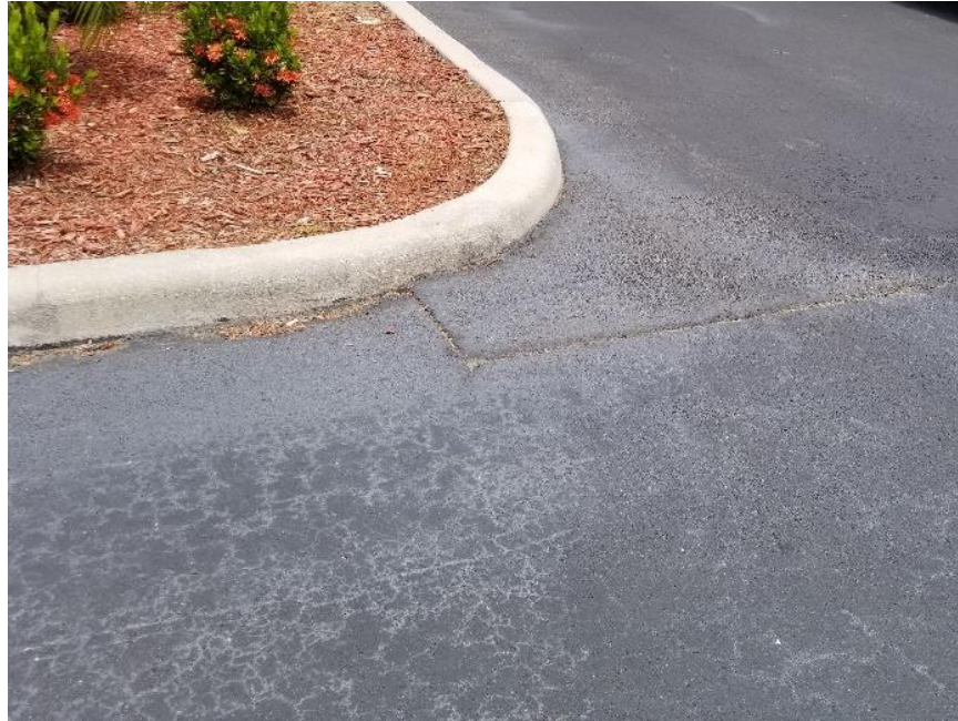
Alligator Cracking and Raveling in Drive (Typical)
